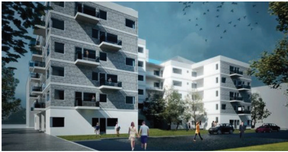
Q KUNGSMYNTAN apartments, Orebro, Sweden
