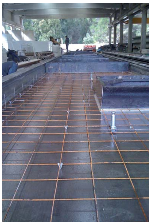
Positioning of supports and knurled connections in the panel.
