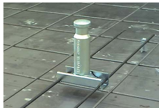
Fig. 1 The support is anchored to the reinforcing mesh of the hanging layer.
