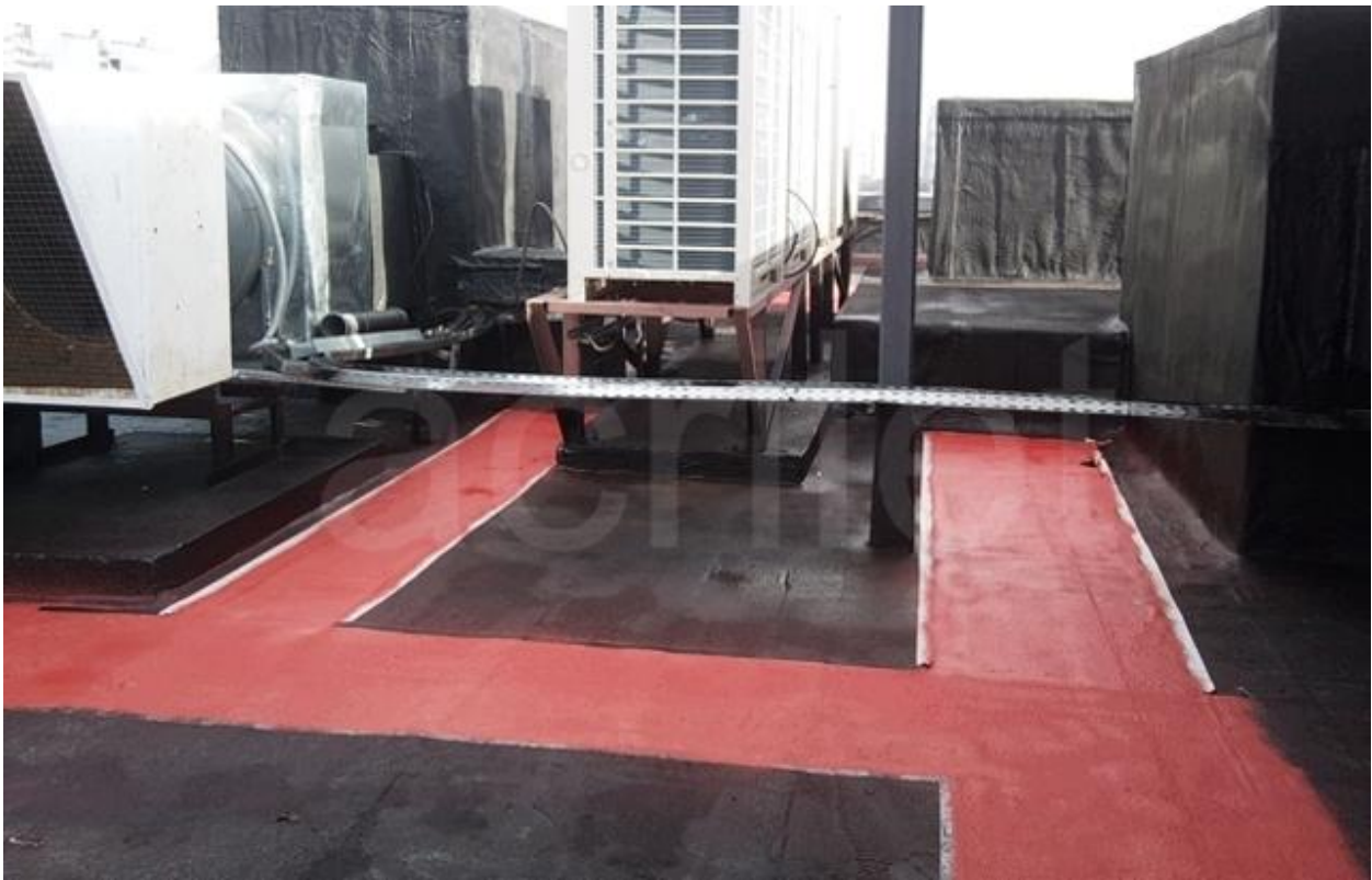
Pathways on roofing made of liquid rubber for equipment maintenance
