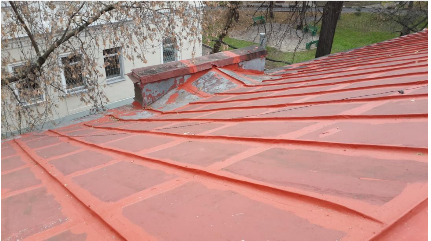
Sealing of frames and metal roofing seams
