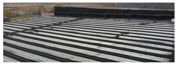
BITUPREN 100 is a bitumen-polymeric mastic used for all kinds of anticorrosive protective treatment of any building structures constantly exposed to UV, water, most of acid and alkali solutions, oxidization and aging. Can be applied on any surfaces such as ferrous and galvanized metals, concrete, slate, wood etc.Easy application and quick drying time make BITUPREN 100 an ideal versatile product for professionals and for those who do their work in DIY (do it yourself) way.
