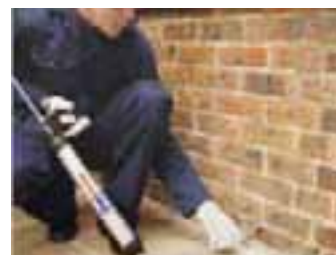
❸ Injection of waterproofing gel.
