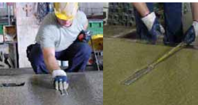
Preparation of guide rail after concrete placement.
