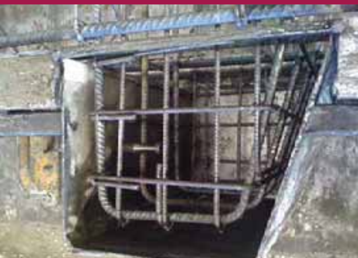
PREPARATION OF RUR BUSHING IN FORMWORK.
