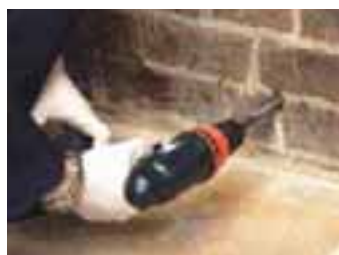
❶ Drilling of holes to be injected with distance and length shown in the table (see below).
