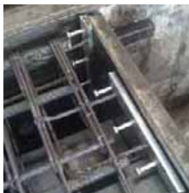
Preparation of guide rail before concrete placement.
