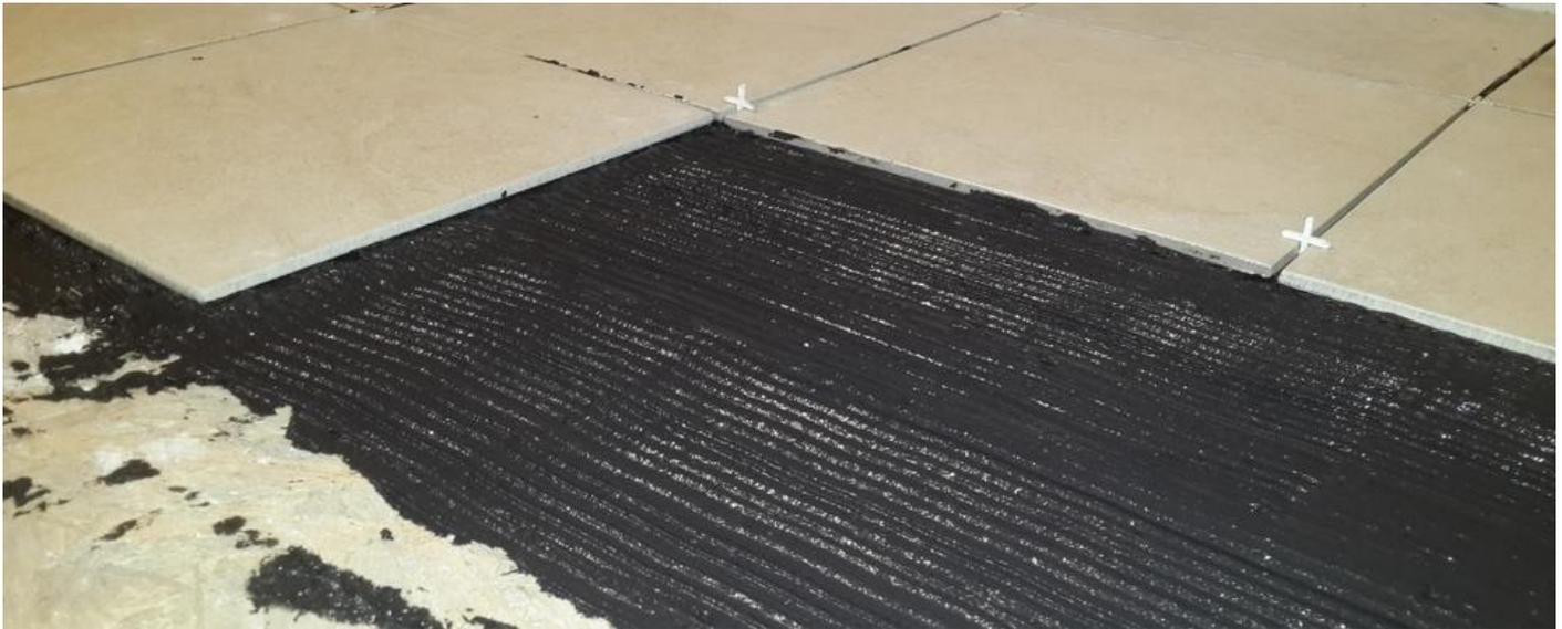
BITUPREN 200 is the latest product designed for reinforcement and cost reduction of the process of tile paving in such areas as bathrooms, basement floors, balconies, terraces and any other places where the surfaces should be protected from water and moisture penetration. The appliance of bitumen-rubber tile adhesive BITUPREN 200 allows paving tiles and waterproofing the floor at the same time.
